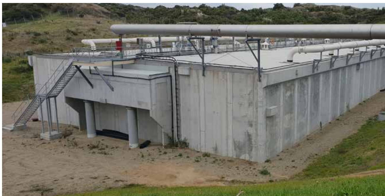
SureLine® HD installation in New Zealand.
