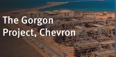
Barrow Island, Western Australia – Gorgon is one of the world's largest liquified natural gas (LNG) projects and the largest single resource project in Australia's history. Gorgon comprises a three-train, 15.6 million tonnes per annum LNG facility and a domestic gas plant with the capacity to supply 300 terajoules of gas per day to Western Australia.
